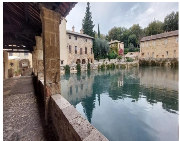
19 Interior loggia and thermal bath
