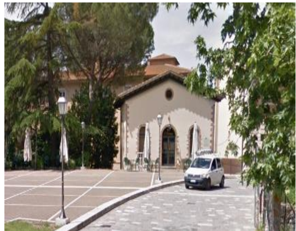
4 Entrance to Hotel Posta Marcucci
